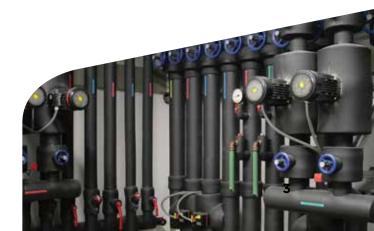
Kaiflex RT-ST Insulated pipe support to prevent condensation and thermal bridges.
